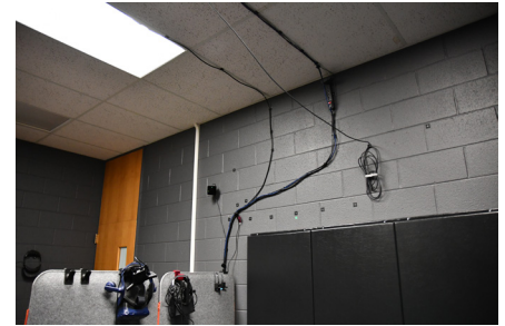
Cables for wired headsets run along ceiling to prevent tripping.
